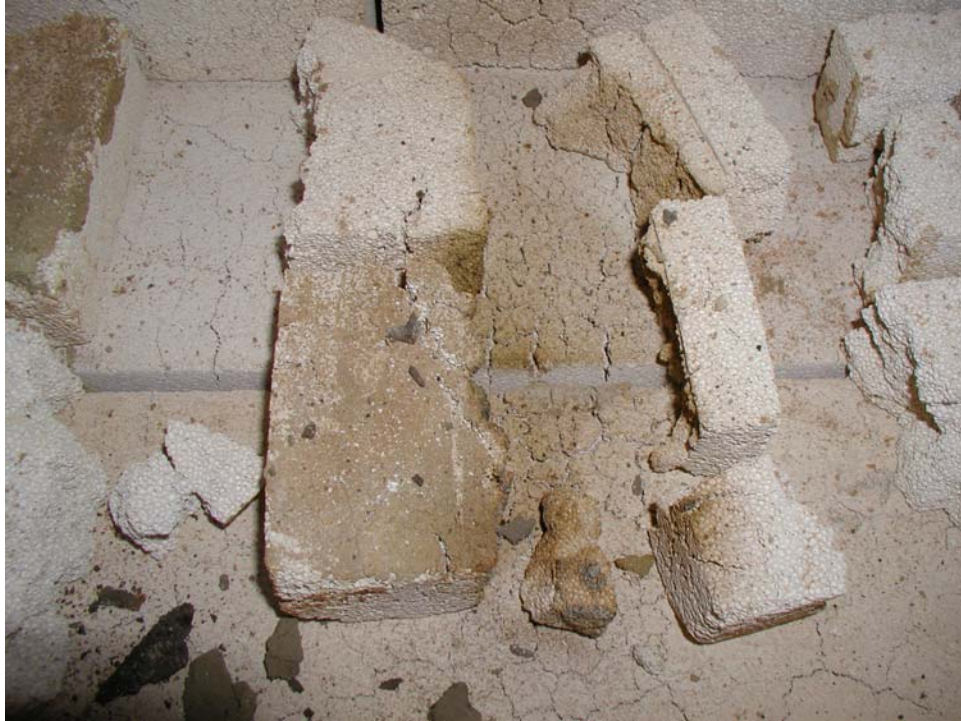
The inside of the kiln after the first firing tells the tale. The Ytong will not hold up to the high temperature.
