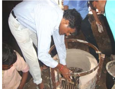
Picture 74 Installation of institutional stove
