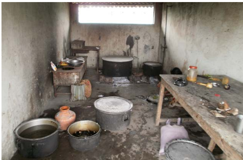
Picture 76 Condition of a Government school kitchen
