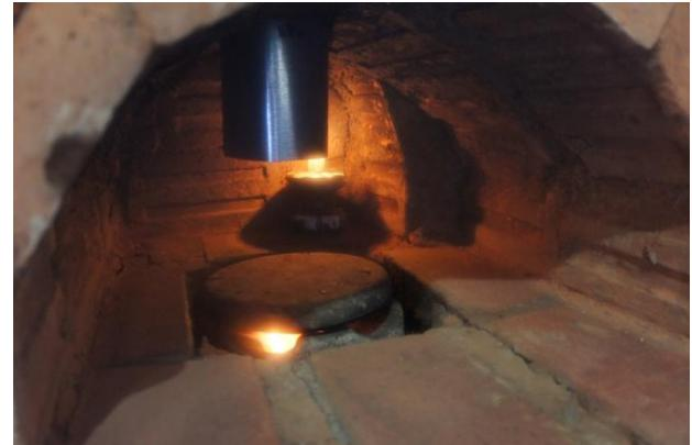
The oven chamber features the holey roket stove beneath the oven floor, a clay disc to deflect the hot gases sideways and unto the walls of the oven, an extended metal cylinder at the chimney. The combination of the two deflectors (the disc and the cylinder) causes the heat to circulate inside the chamber thus give a more uniform and retained heat. My thanks go to Jon and Flip Anderson and Larry Winiarski for the lessons I gathered from their earth oven stove.
