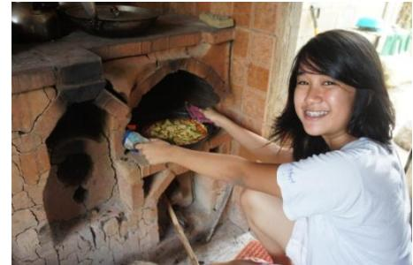
My 4n2 stove oven as planned, built and used. I used mostly bricks that I made and partly I bought at the hardware store. One of the stoves can serve the three cooking ports and the second stove will serve the oven. It took almost three months of drying until we finally inaugurated this project on February 2013 with a very yummy pizza which my daughter Mirasol prepared and enjoyed.
