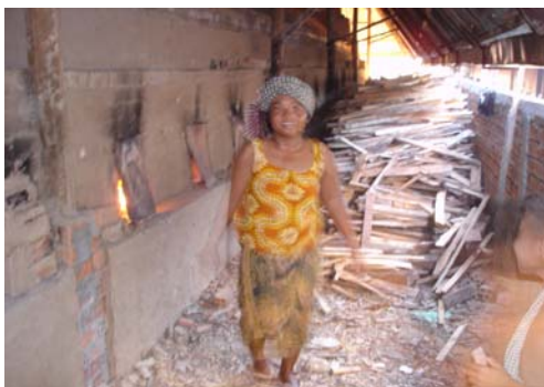
Up: photo of the wood stock in a bricks factory. Down: photo of a worker during a combustion cycle.
