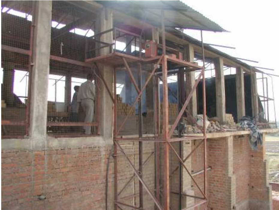
Green bricks are taken to the top of the shaft using an elevator.
