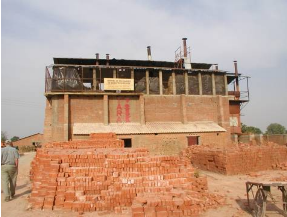
The Development Alternatives Tara vertical kiln near Jhansi, Madhya Pradesh, India. This kiln has three vertical shafts. Each shaft works independently from the others.
