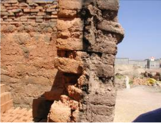
The inside wall of the kiln has become self fired
